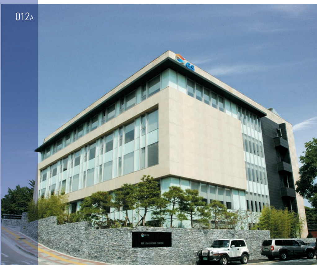
011A Data Center GAK Location: Chuncheon, Korea - Total floor Area: 47,439m 2 - B3 ~ 3F Project Period: 2012. 02 ~ 2013. 06 012A GS Namchon Leadership Center Location: Seoul, Korea - Total floor area: 6,956m 2 - B3 ~ 5F Project period: 2005. 10 ~ 2006. 09
