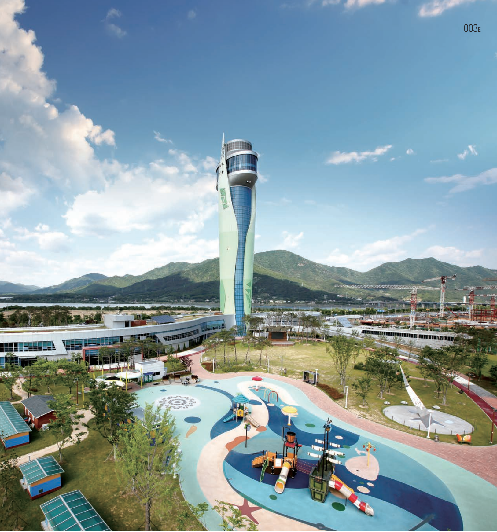
001E Jecheon Municipal Solid Waste Treatment Plant Location: Jecheon, Korea - Incineration plant: 50 ton/day - Stoker type Project period: 2006. 03 ~ 2008. 08
