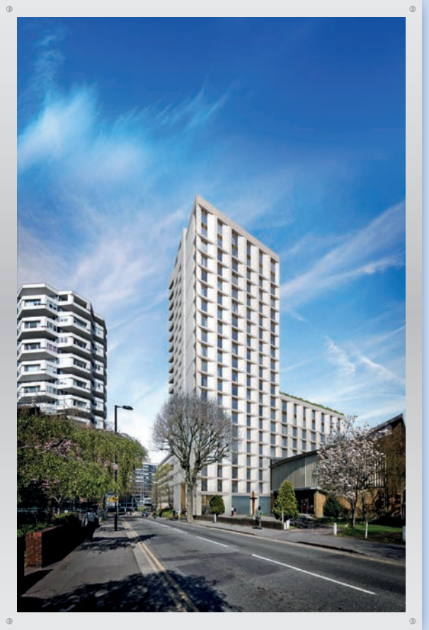
Croydon (21F, London) constructed by Elements Europe Ltd.
